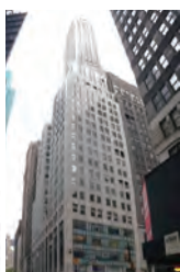
THE AIRSTAGE ON BROADWAY Fujitsu General Solution Center
