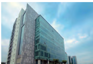
ABS Aircon Engineers Private Ltd. (Indie)
