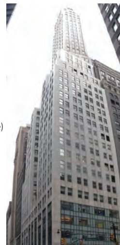
FUJITSU GENERAL SOLUTION CENTER "THE AIRSTAGE" (Stany Zjednoczone)
